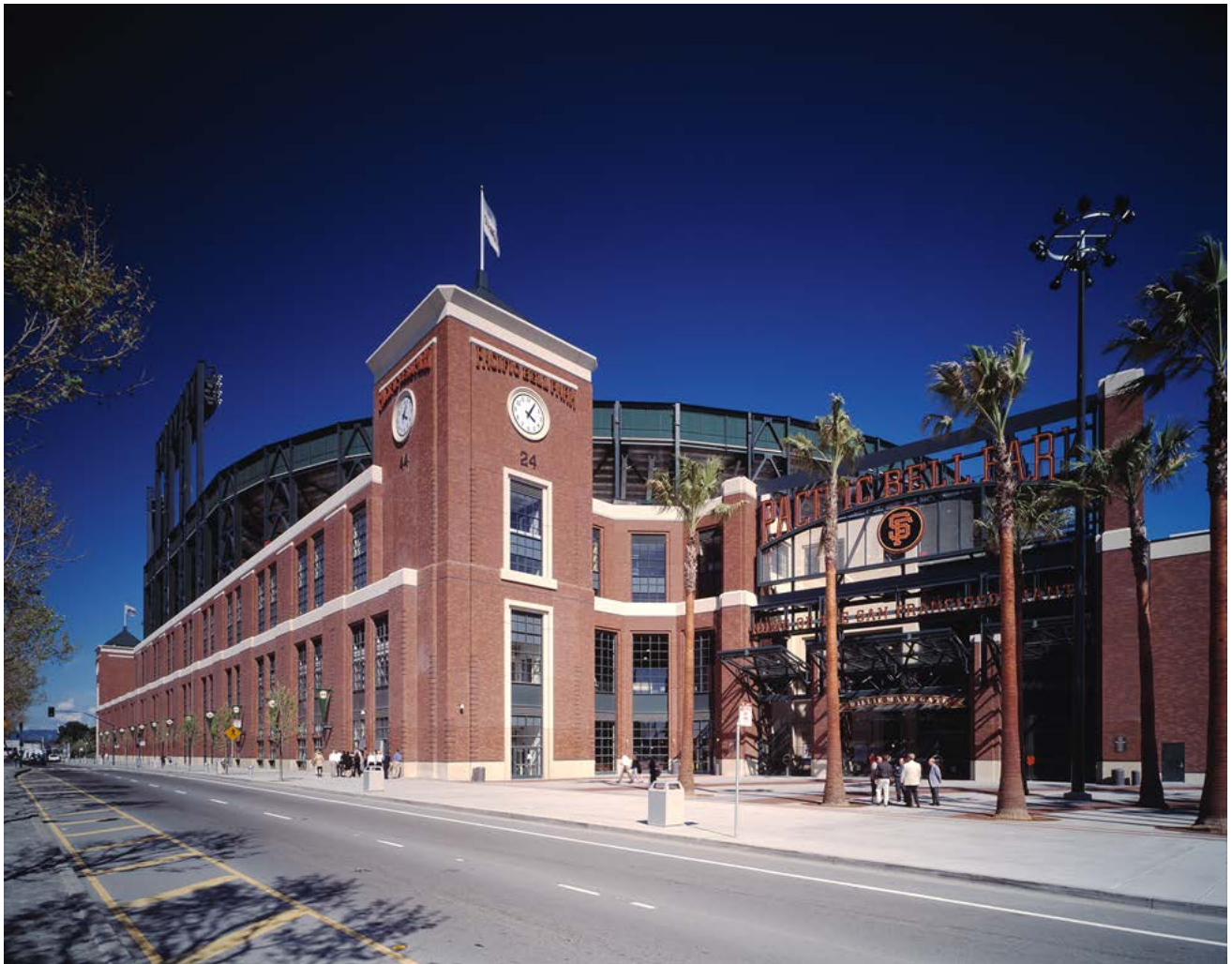
AT&T Park in San Francisco, CA Exterior façade panels brick on precast made in our San Juan Bautista plant.
